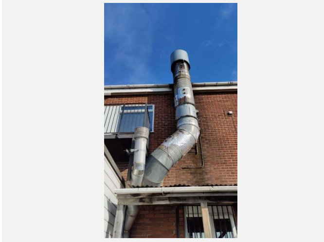
Discharge Ductwork Pre Cleaning
