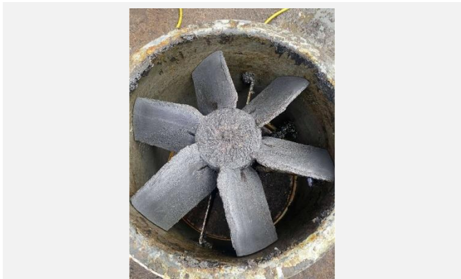
External Riser Pre Cleaning
