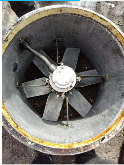
Discharge Ductwork Post Cleaning
