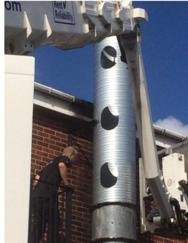
Discharge Ductwork Post Cleaning
