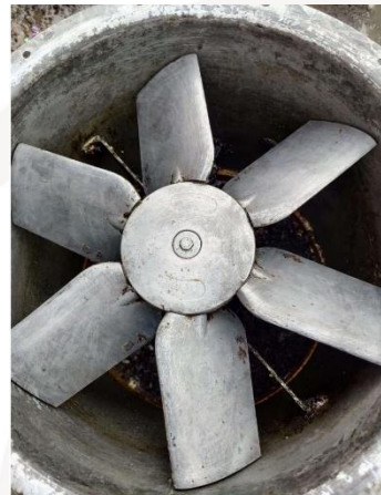
External Riser Post Cleaning
