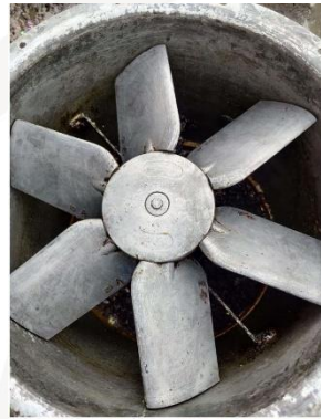
External Riser Post Cleaning
